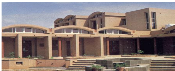
Fig.1 National Institute of Solar Energy located in Gurgaon Region of Haryana (India)
