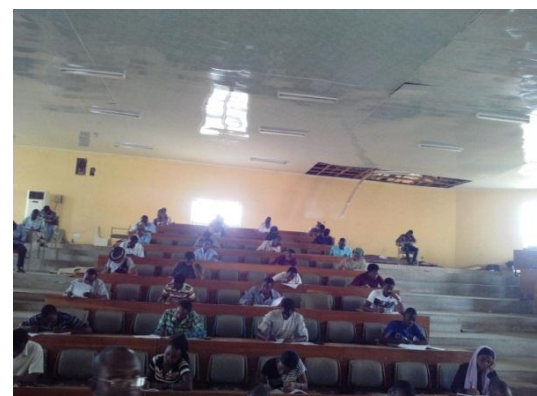
Figure 2.4 Interior of Electrical Eng'g Theater
