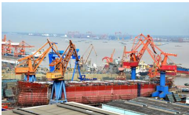
Fig. 3: Example of hull erecting
