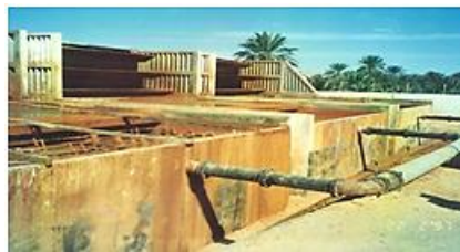
Fig.2 Drilling El Ain Kebili
