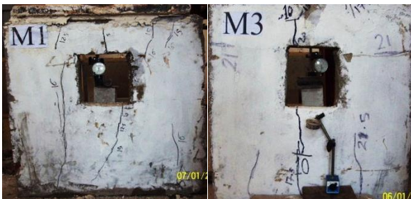
Figure 2 Crack Pattern of M1 Figure 3 Crack Pattern of M3
