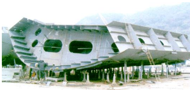
Fig. 2: Example of Block assembly
