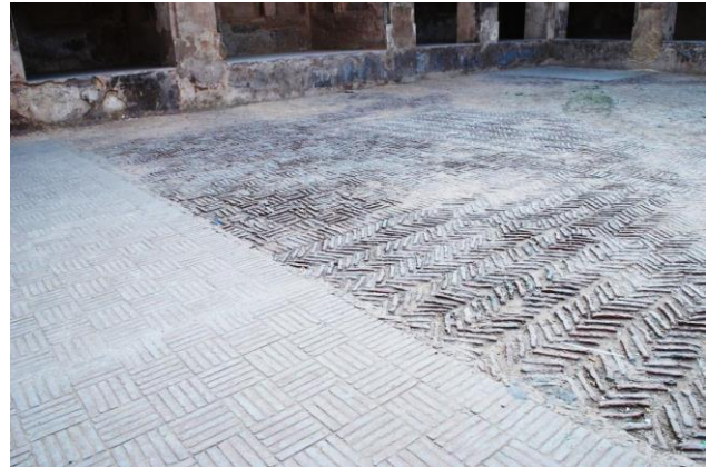
Plate.7 Partly preserved and restored brick soling of floor
