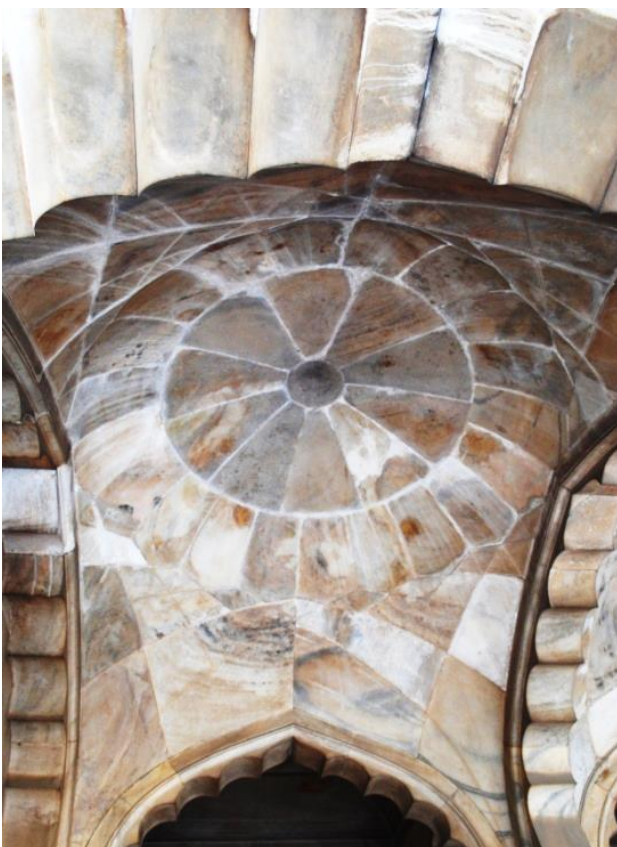
Plate.18 Geometrically lined stones, Interior view looking at ceiling span
